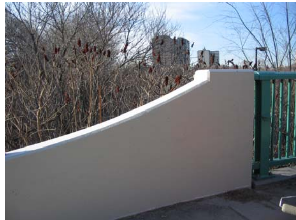
Riverdale Footbridge 'after'
