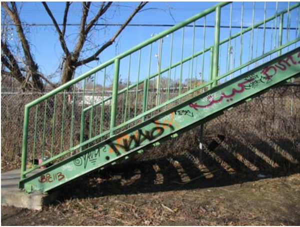
Riverdale Footbridge 'before'
