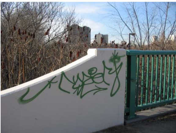
Riverdale Footbridge 'before'
