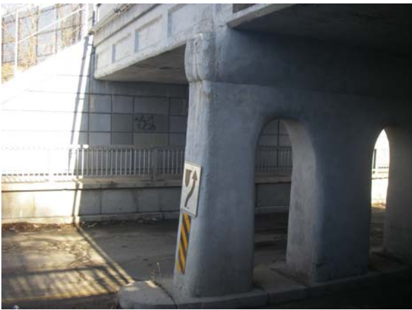
Ray underpass 'before'
