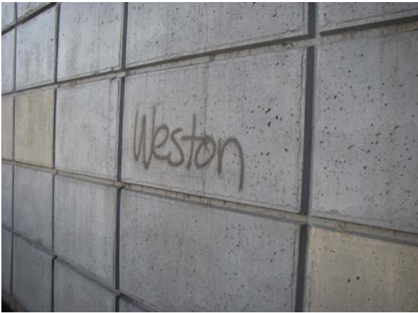
Ray underpass 'before'
