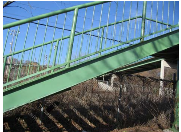
Riverdale Footbridge 'after'
